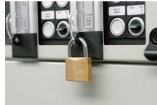
Withdrawable units can be locked in the withdrawn position (up to 3 locks)
