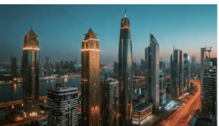
Municipal Utilities & Power Distribution
