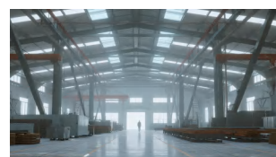
工厂建设 Industrial Plant Construction
