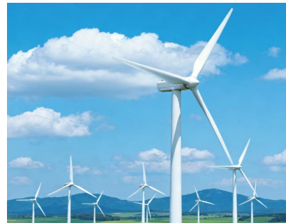
Wind power generation
