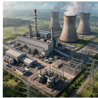
发电厂 Power Plants
